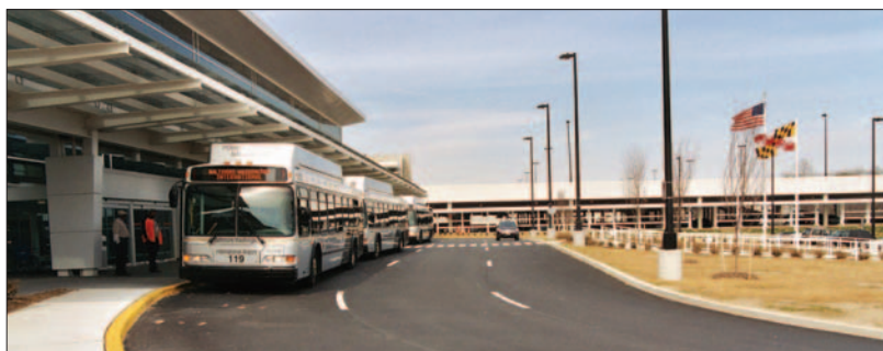
Natural gas-powered parking shuttles are a high-visibility way for airports to reduce emissions while publicly demonstrating commitment to environmental stewardship.
